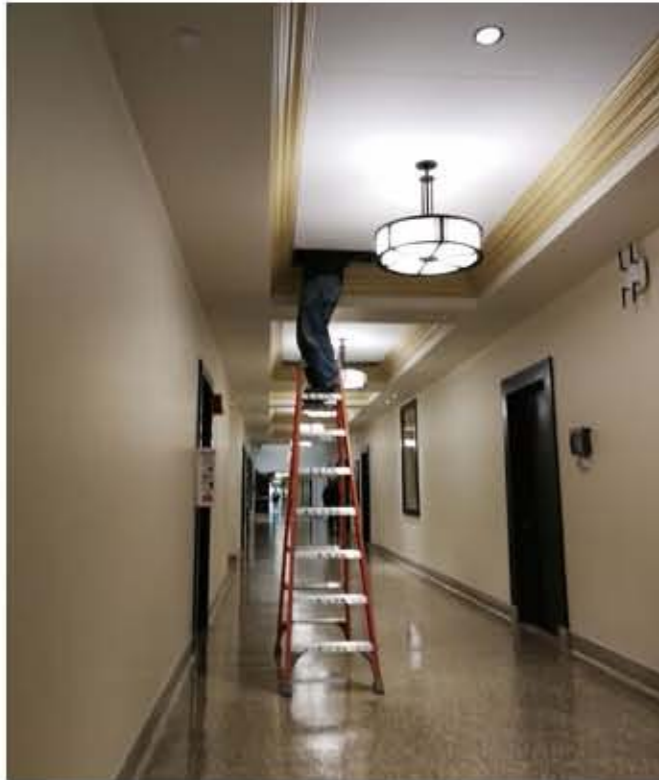
Photo 1 Maintenance task using a ladder
